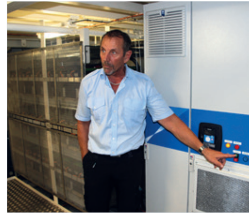
Søren Adersen explains the power conversion system which uses a VACON® NXC Air Cooled microgrid converter. The battery bank is on the left.
